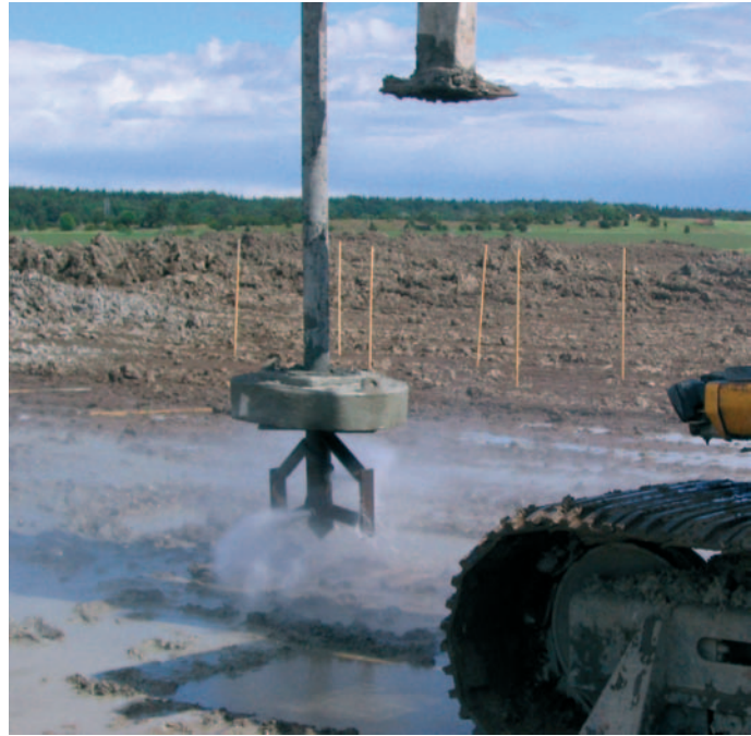
MDM uses modified dry mixing equipment with pressure-sensitive valves to control water injection during mixing.
